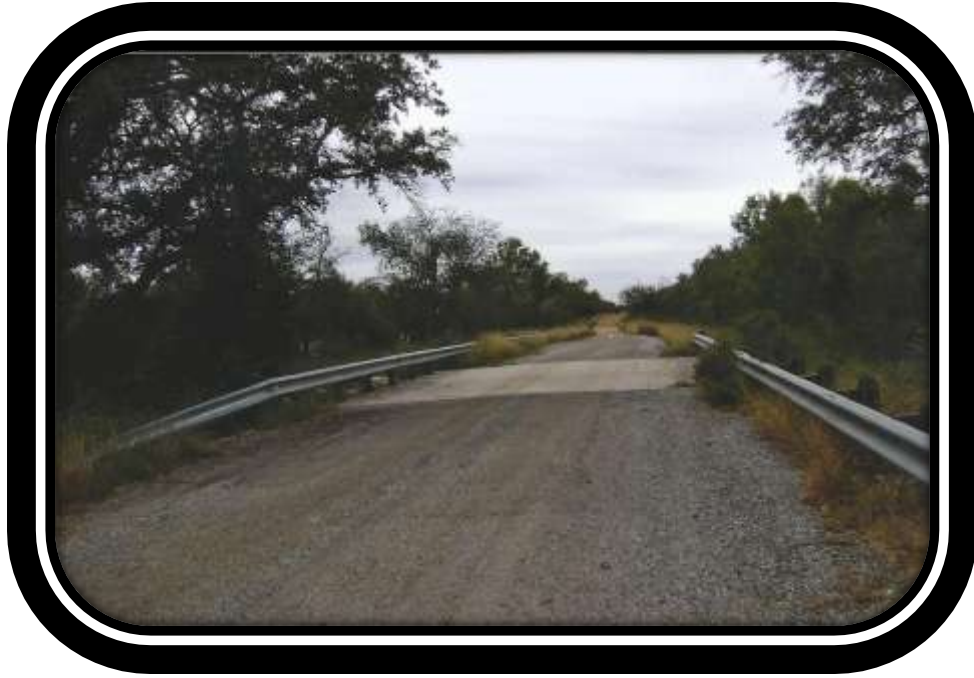
The bridge over Pendencia Creek
